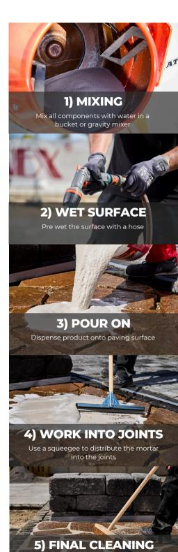
Allow the surface to partially air dry before final brooming
